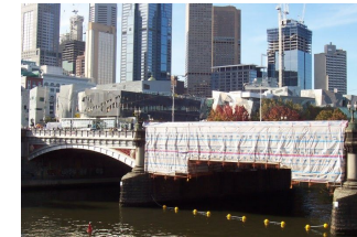
Princess Bridge Princess Köprüsü
